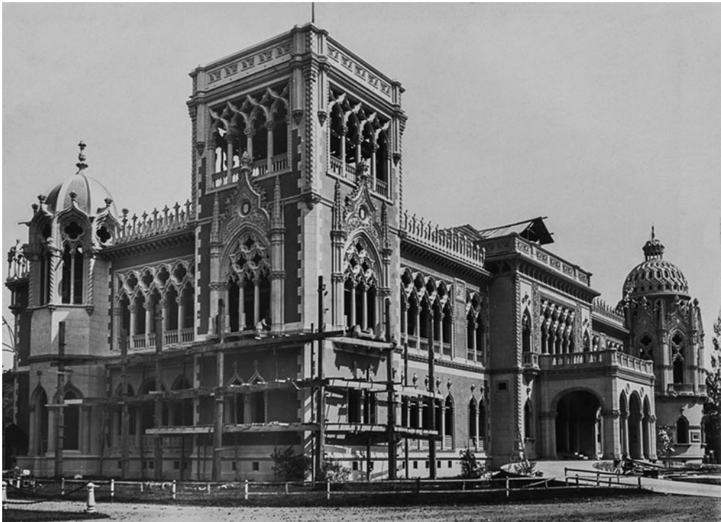
Figure 5. Villa Norasingh in construction (1926), today Thai Government House.
