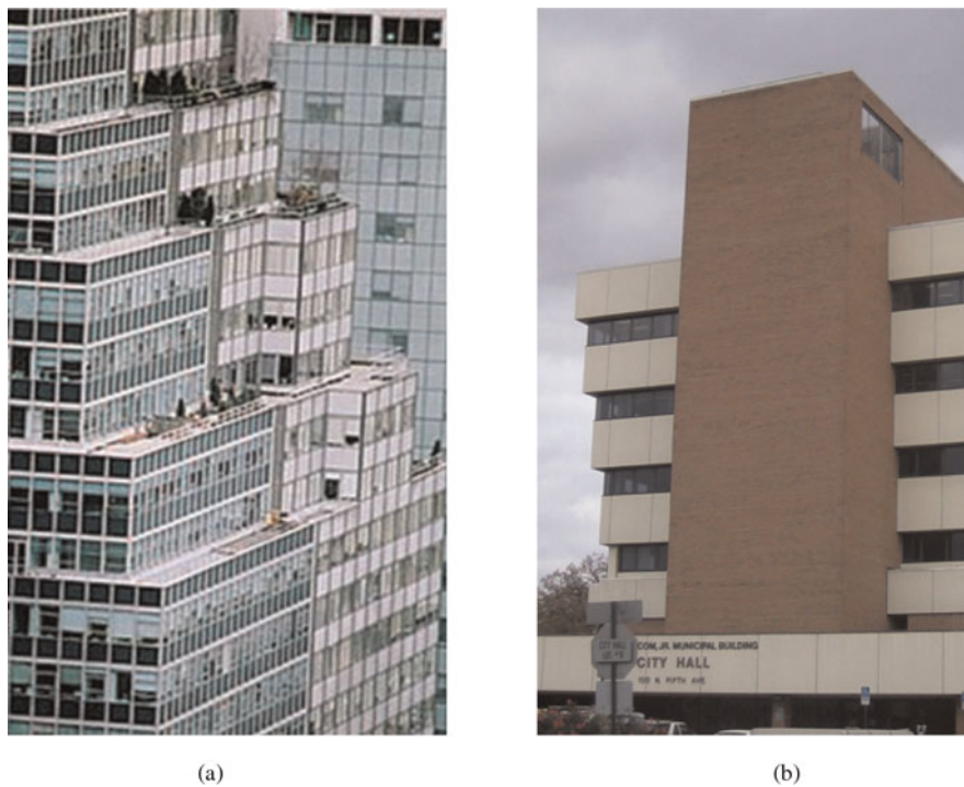
Fig. 1. A comparison of the “stacked” building construction: (a) a traditional form, which is commercial building from Jeff Klamer Design, and (b) a “flipped” form, which is the Ann Arbor, Michigan, City Hall Building. [A color version of this figure can be viewed online at journals.cambridge.org/aie ]
