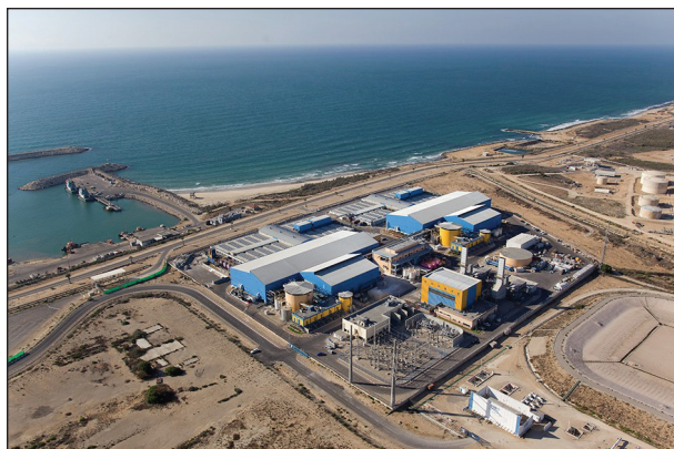
IDE Technologies seawater reverse osmosis desalination plant in Ashkelon, Israel, which has delivered more than 1 billion m 3 of high-quality tap water since the start of operation in 2005.
