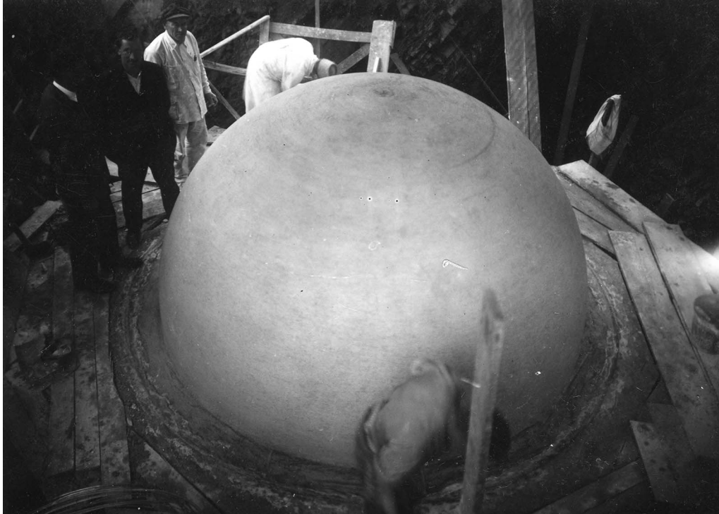
Figure 9. Construction of the underground cave for the ‘Unknown Soldier’ in 1918.
