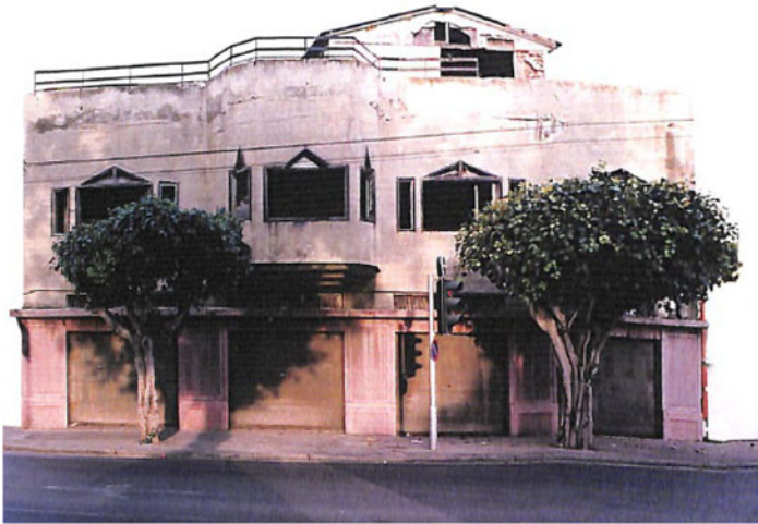
Figure 4. The Arab Library in Jaffa (picture taken in 1997). Tel Aviv-Jaffa Municipality, Archive of Engineering Administration, Building File no. 3000/005, p. 17.
