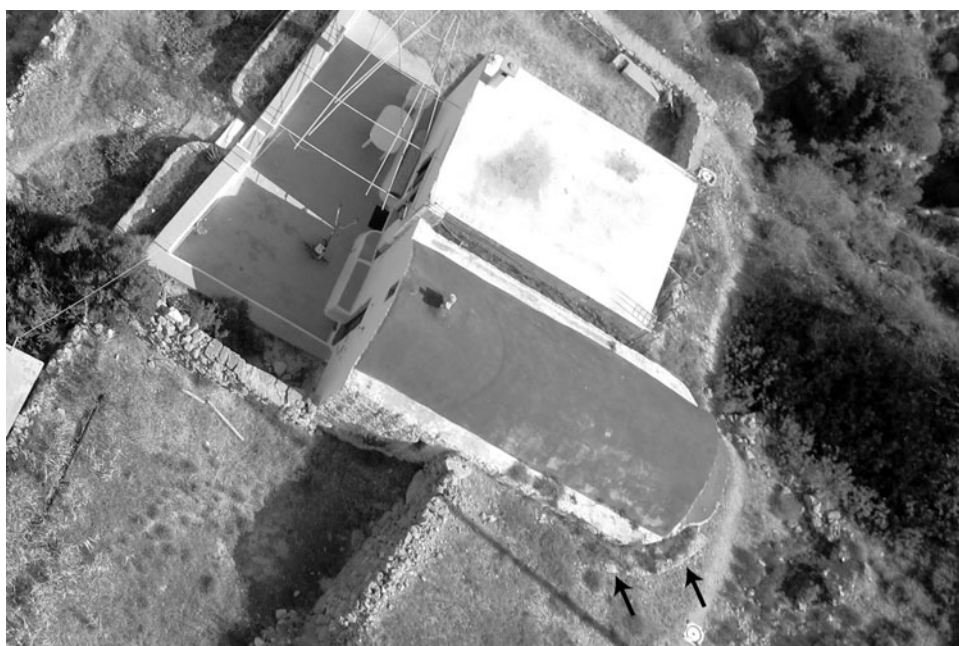
Fig. 19. Aerial photograph of the church of Aghia Panayia Gualo Chorafitissa with apse wall of Early Byzantine church (arrows).
