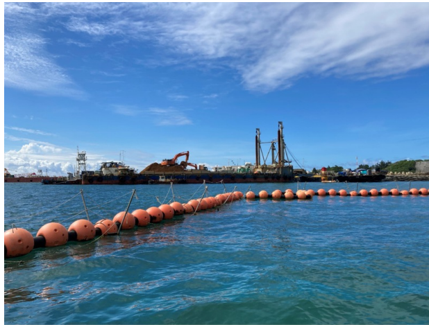
At the construction site in Ōura Bay, © Palz 2021. Every weekday ships and trucks bring soil for landfill.
