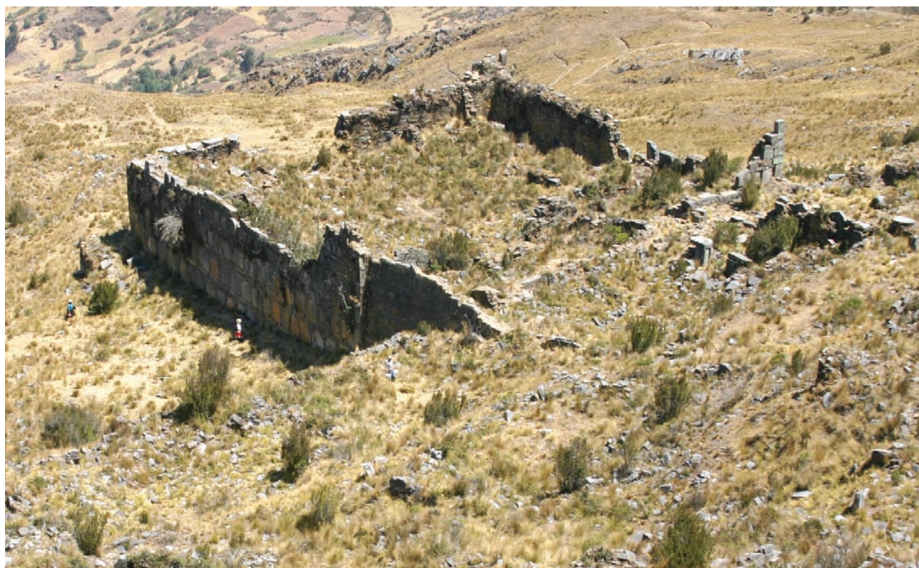
Figure 9. Quadrangular compound c41 (left), view from northeast. The construction rests on a basal platform; a corner can be seen at the middle left. The east façade features at least seven rows of large stones (wankas) set atop narrow, horizontal slabs. The effect is heightened by use of differently coloured granitic and limestone blocks. Directly abutting the building is another compound (c40), featuring a megalithic entranceway into the central courtyard.
