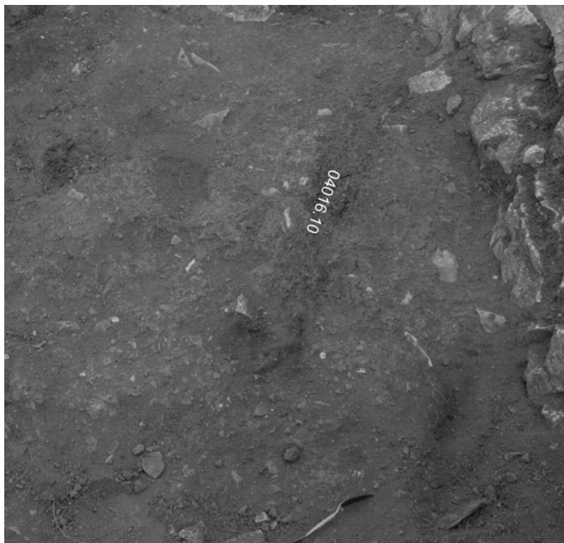
Fig. 27. Building MG1: fallen beam 04016.10 and beam fragments in deposit 04016 from northeast.
