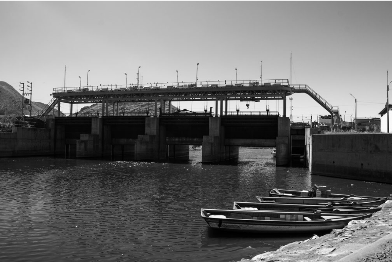
Figure 6. Dam at Desaguadero. (Photograph: S.C. Smith.)
