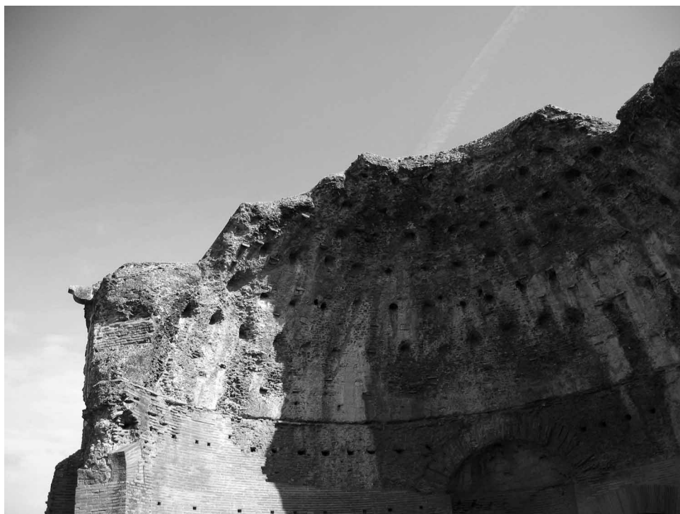
Figure 18. The remains of the dome of the piscina calida at the Heliocaminus Baths. Fragments of the brickwork covering of the intrados are still in place. The hemispheric dome has a diameter of about 12 m at the spring of the vault.
