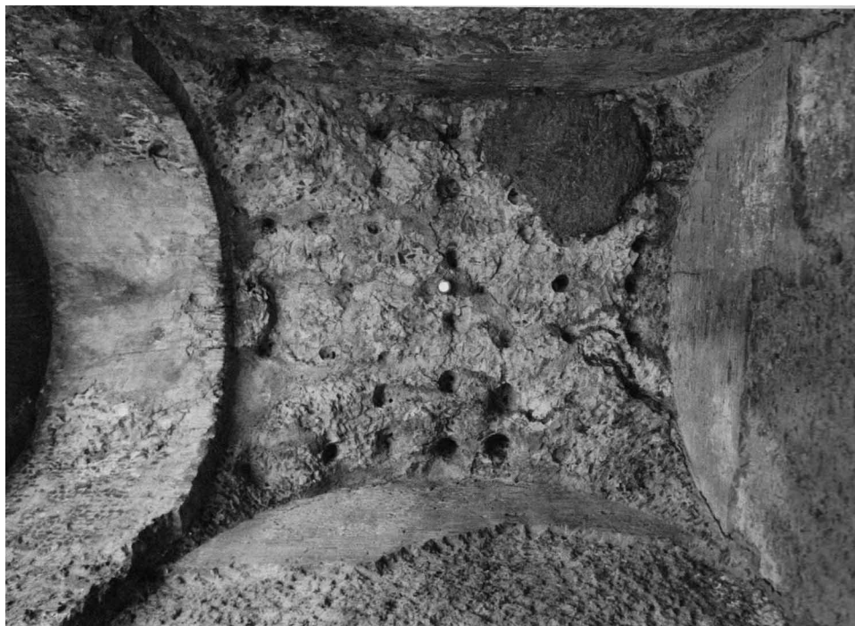
Figure 16. Small Baths in Hadrian's Villa, view from below of the vault of the calidarium number 3, heavily restored. The holes left by the removal of the metal bars are clear. The vertical pipe in the middle of the vault allowed for the discharge of fumes.
