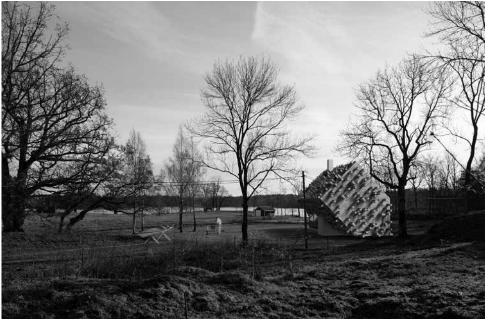
11 Rusticus Dalslandsstugan 2.0, view of Upperud proposal, 2015, Brrum in collaboration with servo stockholm.
