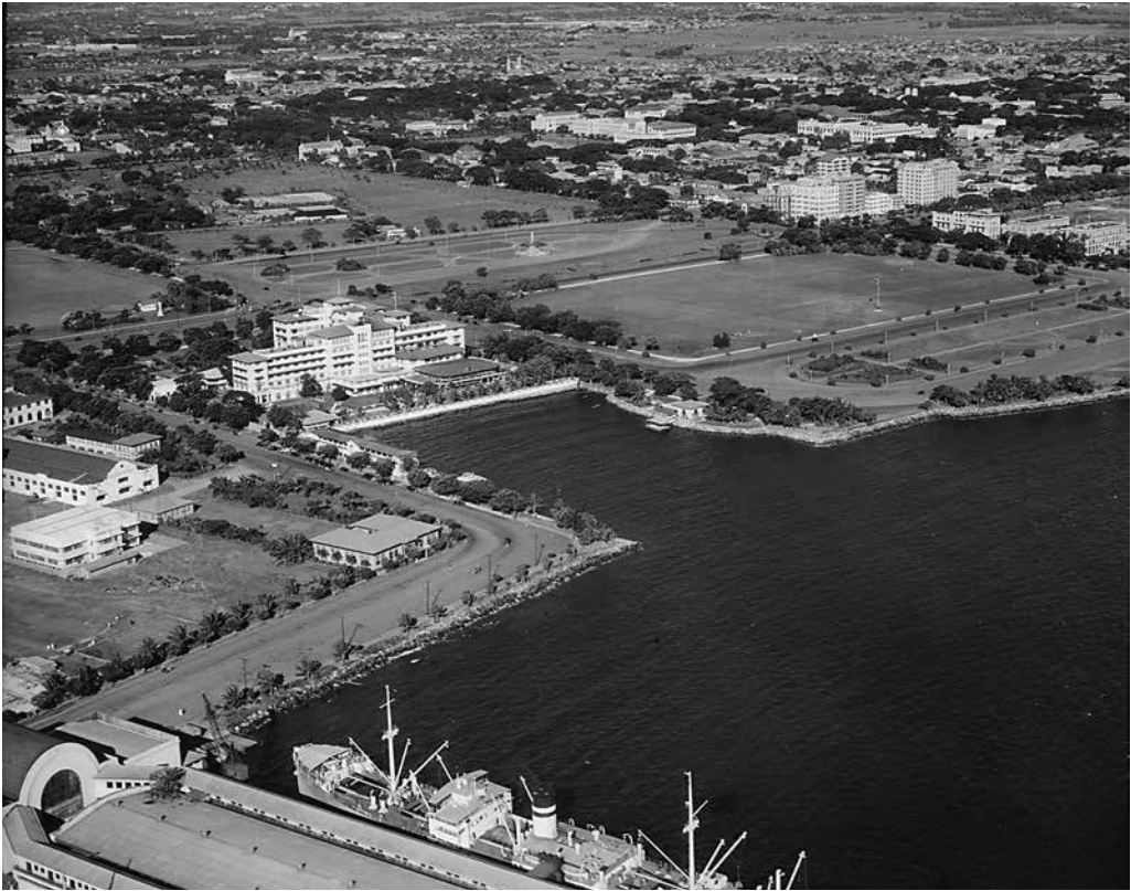
Fig. 7. The Luneta, Manila, aerial view from the west, photograph by George M. Tweedy of US Army Air Corps, 1938. William E. Parsons's Manila Hotel (1912) in the foreground faces his Army and Navy Club (1911) across the plaza (National Air and Space Museum, Washington DC)
