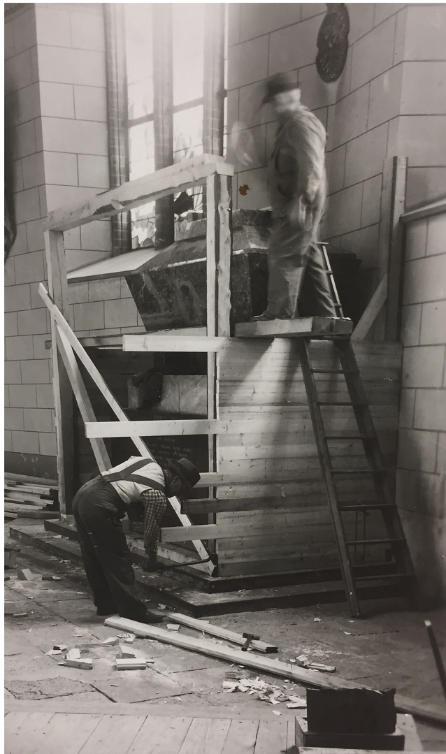
Image 1. A protective structure is being built around the tomb of King Erik XIV in Västerås Cathedral, April 1940. Courtesy of Västmanlands Läns Museum, Vlm-A 658. Photographer unknown.
