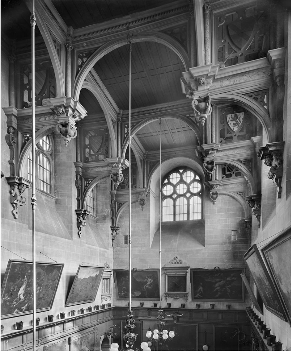
Fig. 12. The roof of the great hall at Wollaton Hall, Nottinghamshire (built 1580–88; © Country Life). The hammerbeam trusses are decorative rather than structural, as there is another chamber (the 'Prospect Room') above the hall. The roof may have been influenced by that of the great hall at Theobalds
