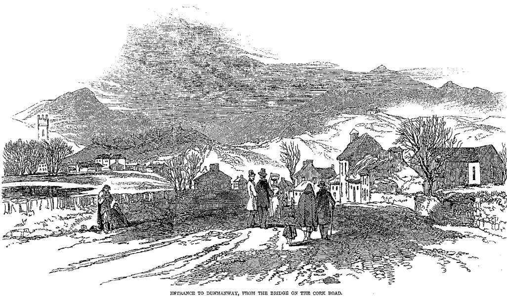
ENTRANCE TO DUNMANWAY, FROM THE BRIDGE ON THE CORK ROAD.
