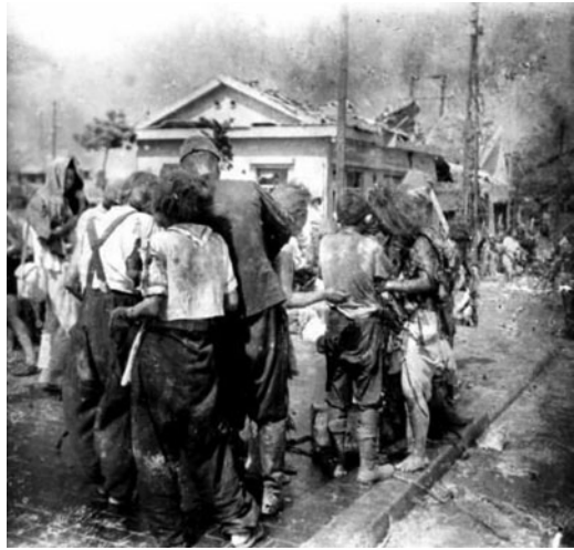
Figure 2. West End of Miyuki Bridge, 2.2 kilometres from the hypocentre. Survivors suffering burns receive dabs of cooking oil brought from the Hiroshima Army Provisions Depot nearby, or oil used for the transformers of the Hiroshima Electric Railway. Photo by Yoshito Matsushige, © Chugoku Shimbun .
