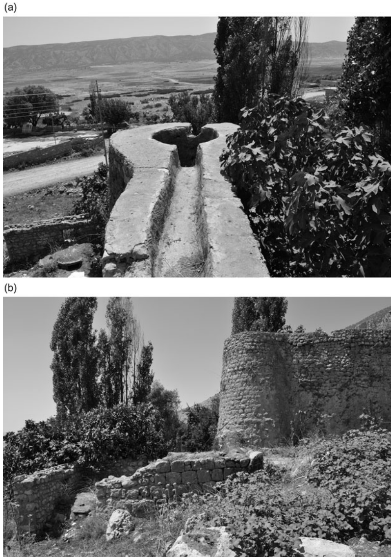
Fig. 15 a) Channel bringing water to the gristmill drop-tower (note the opening in the cylindrical holding-tank); b) channel, drop-tower and millhouse, Yekmala (site 315). © LoNAP
