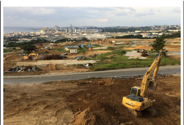
Construction work to remediate land at Nishi-Futenma, Okinawa
