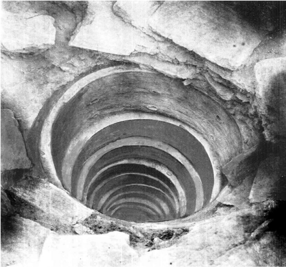
Fig. 1 Early Dynastic period ring-drain at Khafaje, Temple Oval M 44:8 (from Delougaz 1940: 124 fig. 113). The cap is missing, affording a view down inside the drain
