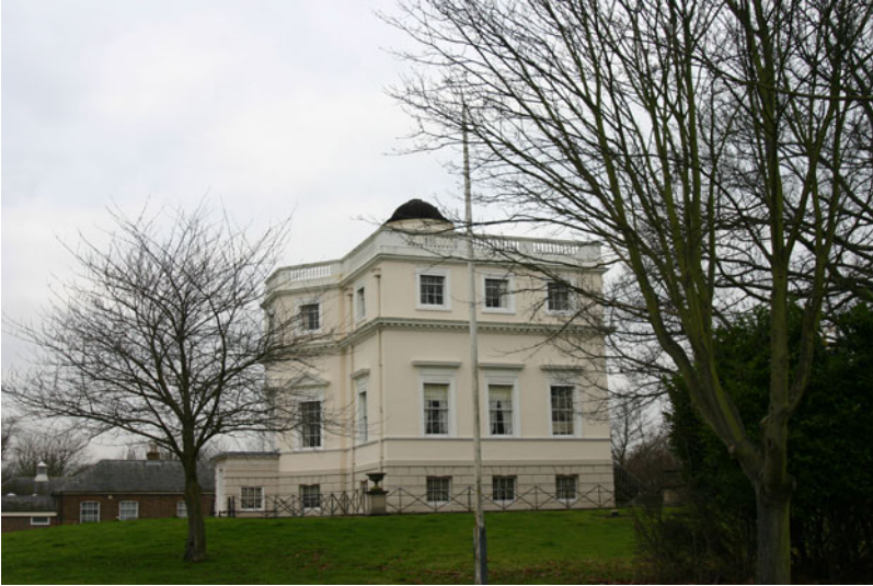
Figure 1. Kew Observatory, photographed by the author in December 2012. At the time of writing (early 2014), the building is unused and in the hands of a property developer.
