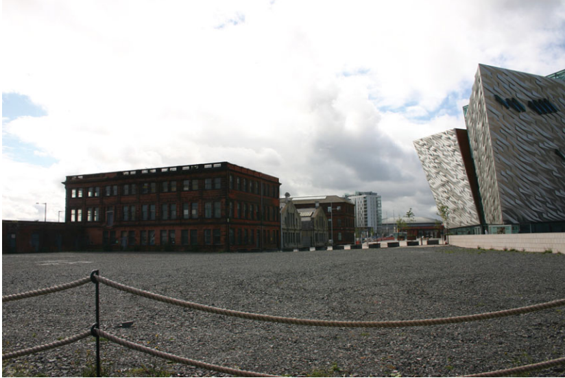
Figure 1 Derelict Harland and Wolff drawing offices (left) adjacent to the new Titanic Belfast building (right). Photo by author.
