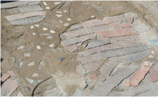
Fig. 25. Imperial Palace, Portus (Fiumicino, Rome), Room 12, detail of the two preparation layers. (E. Gasparini. By permission of the Portus Project.)
