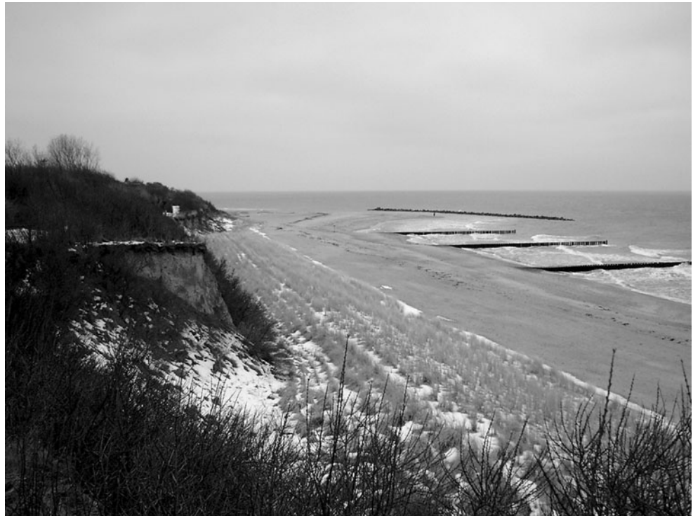
Figure 3 Ahrenshoop, looking south-west, showing the breakwater, groynes and protective foredune designed to protect the bluff but allow it to function as a hinge point and feeder beach for the adjacent low-lying coast. Note the linear artificial nature of the dune at the base of the bluff.
