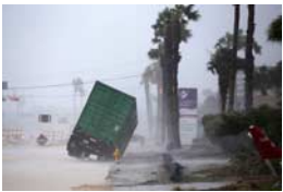
Overturned generator outside hospital during Hurricane Harvey. Source: Google Images.
