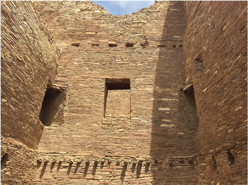
Figure 1. Multi-storey section in the East Wing of Pueblo Bonito (Room 242), Chaco Canyon National Historic Park. This room lies within the last major addition to the 800-room building, a construction episode that dates from AD 1077–1084. Dateable Pinus ponderosa roof beams and lintels in this room were cut between AD 1080 and 1082 and transported to Chaco from surrounding highlands. Two of the building's seven corner doorways lead diagonally out of the second storey of this room to adjacent rooms, which made it one of the most connected rooms in Pueblo Bonito. The height of the ceiling of the second storey from the floor ledge (above the first-storey roof) is 2.9m (photograph by Barbara J. Mills).
