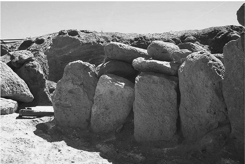
Figure 5. General view of the Tulán-52 structures and detail of a wall with large vertical building slabs topped by horizontal ones. The stratigraphic profile of the mound that covered the site is visible in the background.
