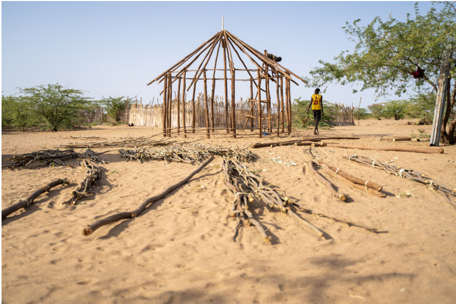
Figure 3. House construction in Nakurio using etirae timber in 2022.
