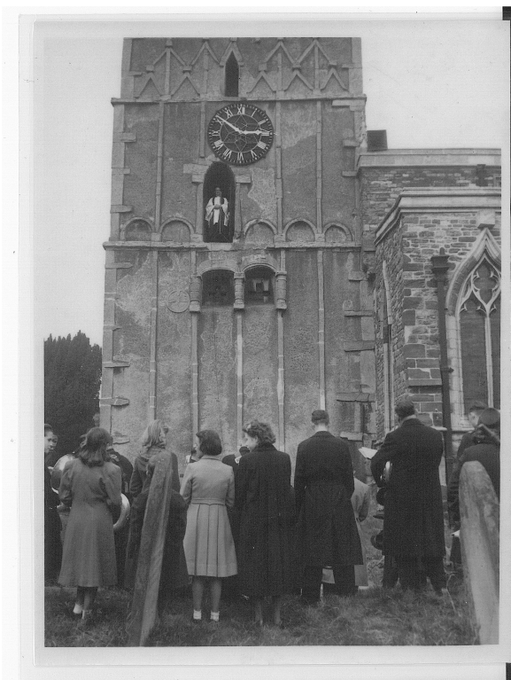
Fig 19. Louis Ewart, Vicar of Earls Barton, delivering a sermon to a crowd assembled in the churchyard of All Saints, 1954. The tower-nave may have been used by the wider community in such a way from its construction in the mid-eleventh century. Photograph: Earls Barton Museum of Village Life.
