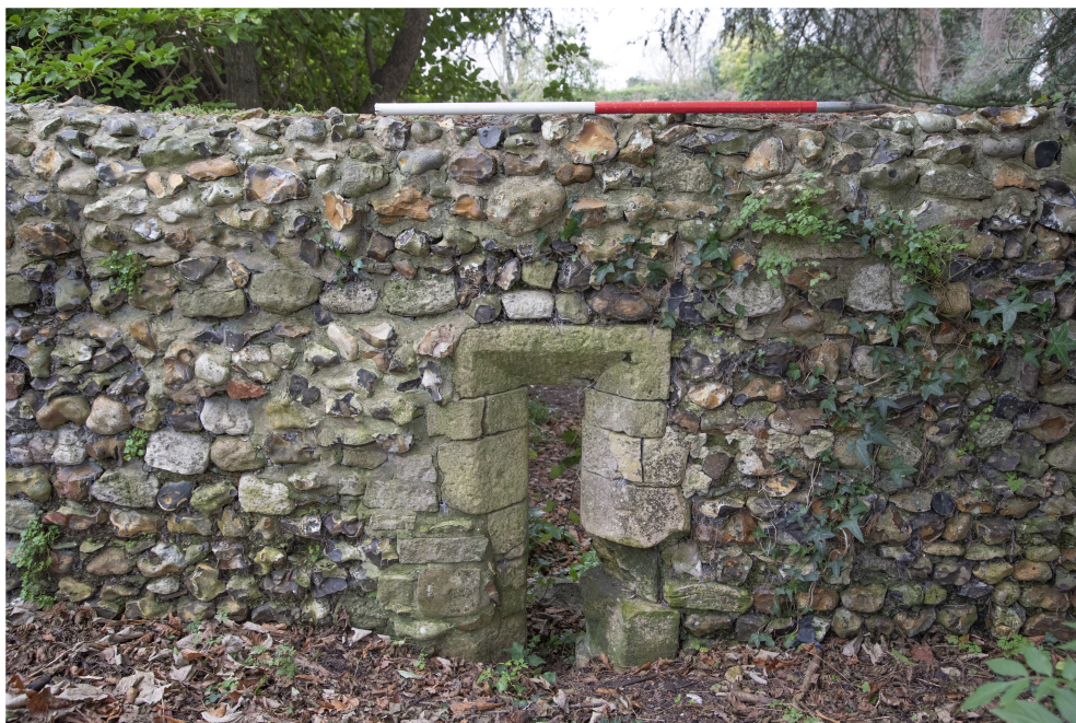
Fig 10. Garden ruin, Bosham Manor House, lancet window to northern half of west wall. External view looking east. Image : authors.
