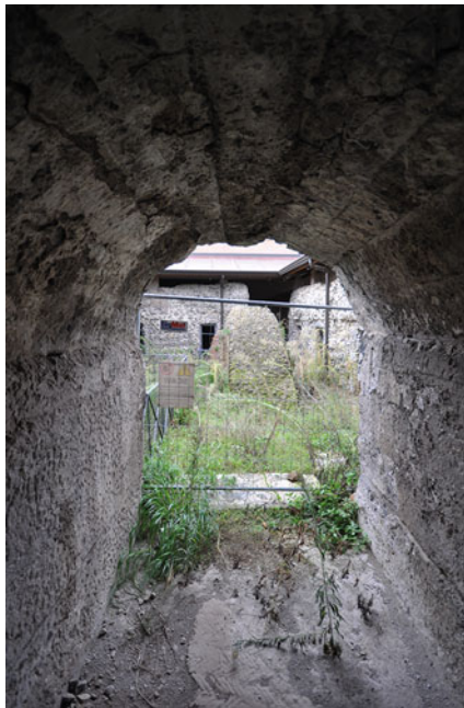
FIG. 5. View from passage 1 into the basement area of the 'house of Livia'; the concrete core of the staircase (Fig. 3 'S') is visible in the middle of the 'Peristylum'. (Photo: Patrizio Pensabene 2021a: 260, fig. IV,24)
