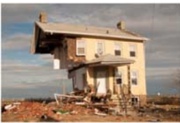
Damage to home at Union Beach, NJ. Image courtesy Patsy Lunch/FEMA
