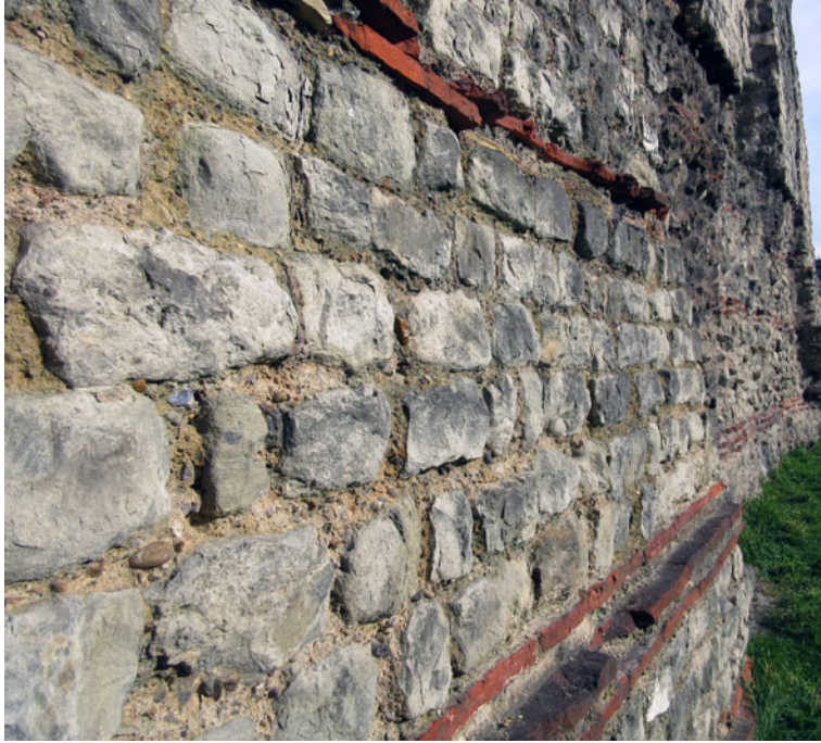
FIG. 4. Detail from the surviving section of the Landward Wall by Tower Hill. The view shows the brick bonding – or lacing – courses arranged at regular intervals with two or three rows of bricks and the angular Kentish ragstone blocks used for the wall's facing (photo by K. Hayward).
