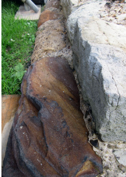
FIG. 9. Basal chamfered plinth in ferruginous sandstone (brown) and Weldon and Barnack limestone (pale-cream/white) from a section of the Landward Wall by the Wardrobe Tower, Tower of London (image by K. Hayward).
