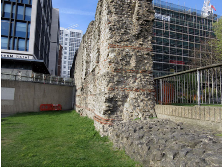
FIG. 2. Surviving section of the Landward Wall by Tower Hill showing the variety and durability of material types, particularly the bonding or lacing courses of Lydion brick and hard angular Kentish ragstone blocks. The Roman remains constitute the first c. 4.5 m of the height of the wall, with the rest being medieval (photo by K. Hayward).
