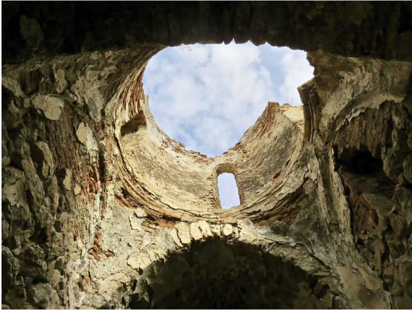
Image 3. The partially collapsed dome of a church within Dêr Meryem Monastery. Author's photo, November 2015.
