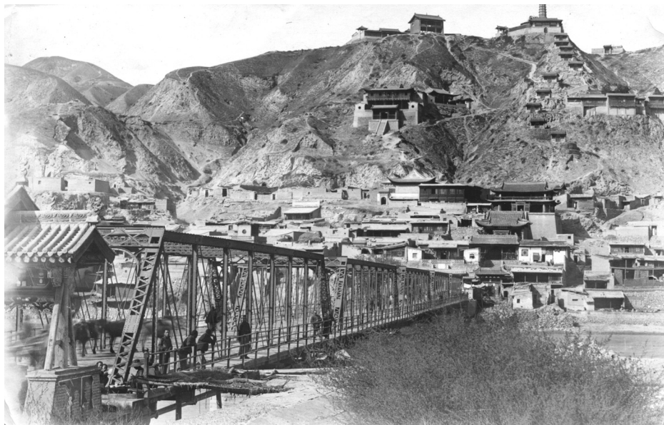
View from Lanzhou to opposite bank of Huanghe River, 1920s/30s.
