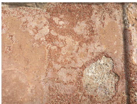
Figure 1. Roman opus signinum from a domestic cistern in Lucentum (Alicante, Spain). Note the remains of the smooth surface (left); smoothing closes the pores, thus improving impermeabilization. Here, the lining was applied on top of a base layer of sand-lime mortar.
