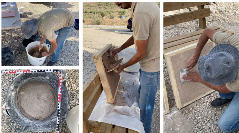
Figure 5. The four main stages of mixing and applying opus signinum.
