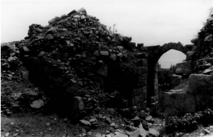
PLATE XVII. ‘Ādilābād Gate, interior of the single straight corridor from the north-west leading to the main portal, also showing a niche in the wall of the corridor to the left, instead of an opening to a gallery which is absent in the design of this gate. There is a corresponding niche on the opposite side.
