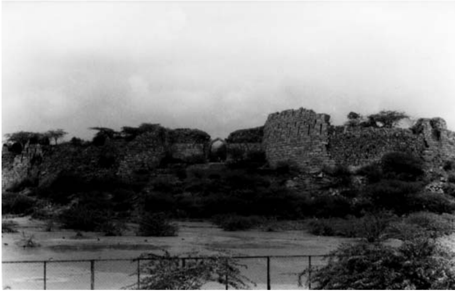
PLATE X. Tughluqabad Town. The southern wall of the town with the Khirkī Gate and the ghāt leading down to the lake.
