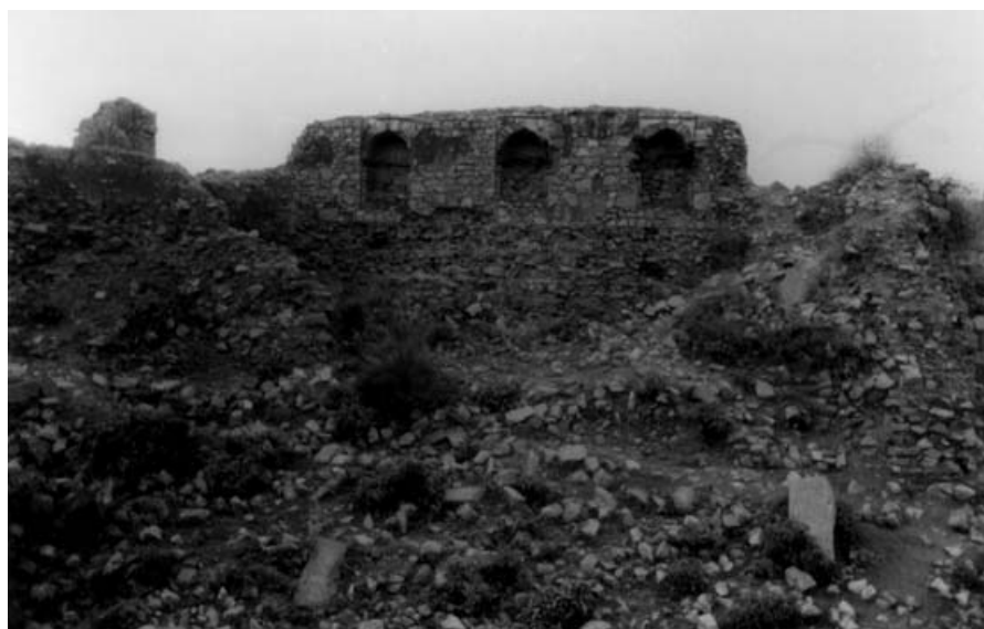
PLATE VI. North Gate, interior seen from the east, with the ruins of the gallery and niches of its western wall side. Although much of the stone has been pilfered, the floor line can still be seen on the wall and part of the original plasterwork is also preserved. In the foreground is the longer portion of the dog-legged corridor.
