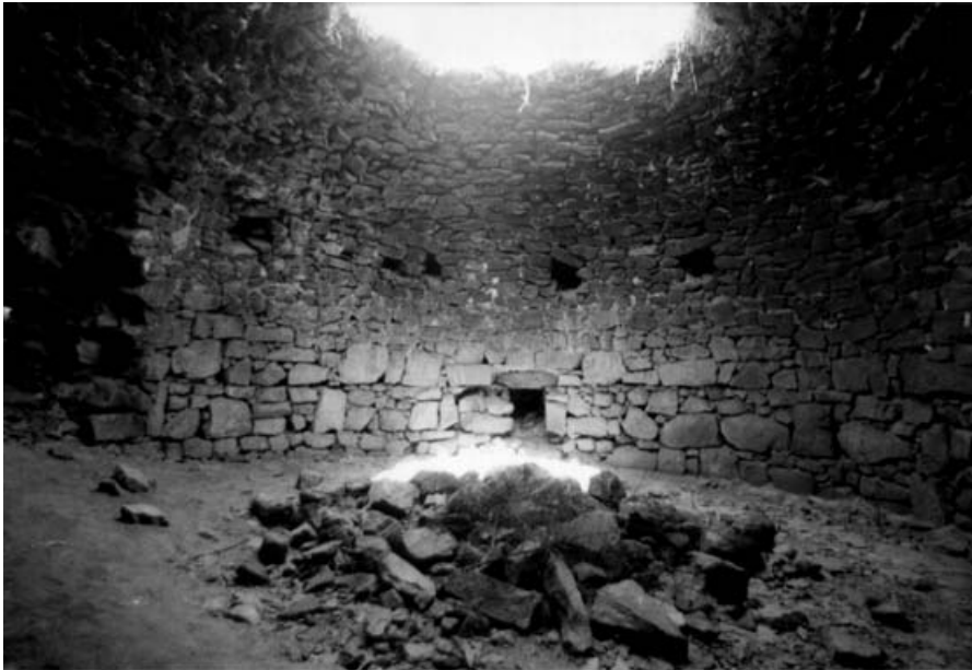
PLATE XIX. Interior of a silo to the north-west of the Hāthī Gate, now filled with debris almost to the springing of the dome. A chute for filling the silo can be seen in the centre, and a row of gaps in the stonework to hold the scaffolding at the time of construction of the dome have not been filled, indicating that a fine finish was not required on the interior.
