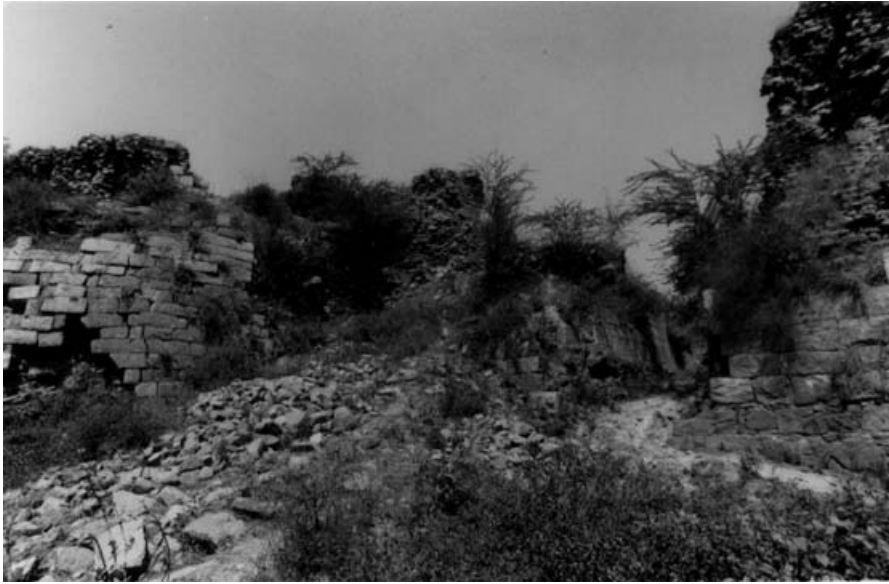
PLATE VIII. Hāthī Gate, remains of the exterior portal with flanking towers which are unusually close to the portal. Through the opening of the portal, part of the sloping corridor and the arched openings to the collapsed western gallery can also be seen.
