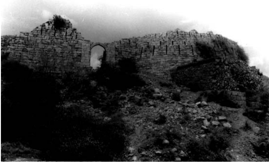
PLATE XVIII. 'Ādilābād Gate, view from the south showing the outer portal, the single tower to its east and ground between the gate and the lake, with the causeway to 'Ādilābād added later to the right. The stonework of the gate—a later addition—does not match that of the tower and the loopholes of the gate are arranged differently, and not at the same level as those of the tower.
