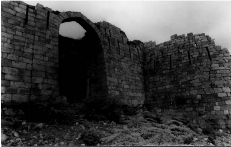
PLATE II. Andheri Gate, view from the south-west looking at the grand portal encasing a smaller arch and the south-east corner tower of the town on the right. The stones of the gatehouse are not keyed in to the tower indicating that the gate would have been constructed after the completion of the tower.
