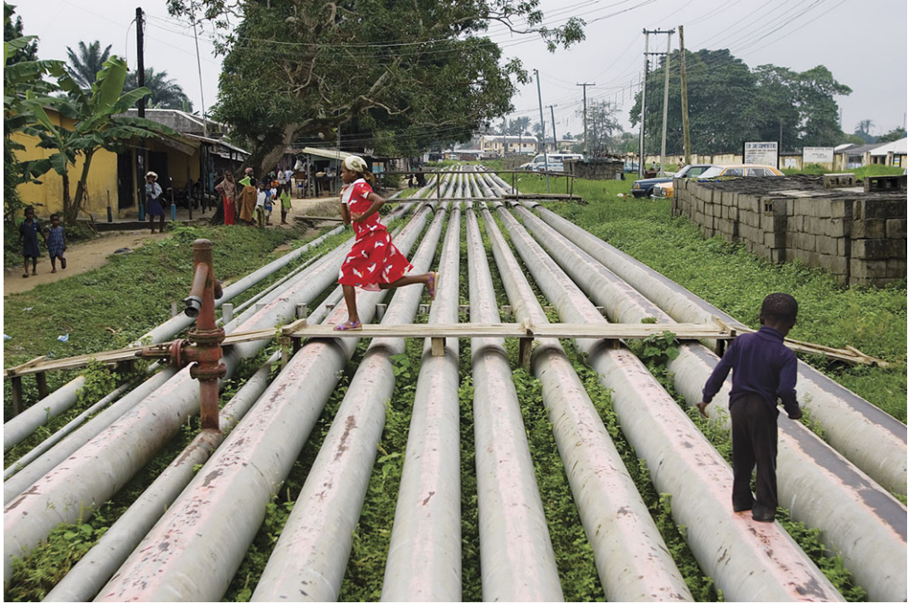
Figure 4: Children play on the oil pipelines in Okrika. This conflict-ridden oil-producing town ten miles to the southeast of Port Harcourt on the Bonny River has experienced oil leaks and oil fires along these pipelines, which run directly through the town on the way to the coast terminal managed by the Nigerian National Petroleum Company (NNPC).
