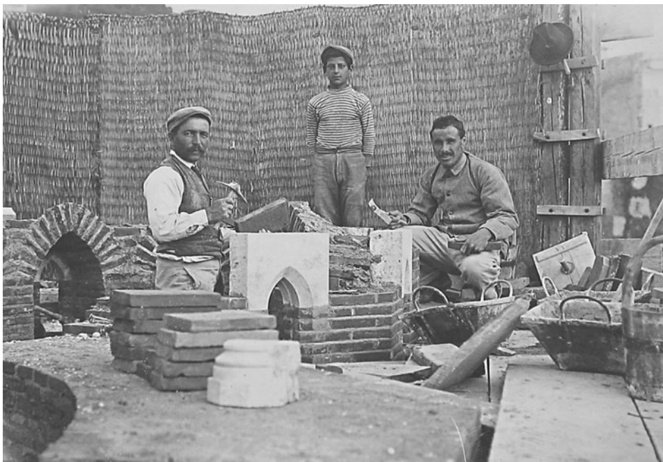
Fig. 6. Rare image of Roman builders (Messrs Maggiorani) erecting one of Street's churches (in this case, All Saints'), c. 1885 (USPG Archive, Bodleian Library, Oxford, C/EUR/Rome).
