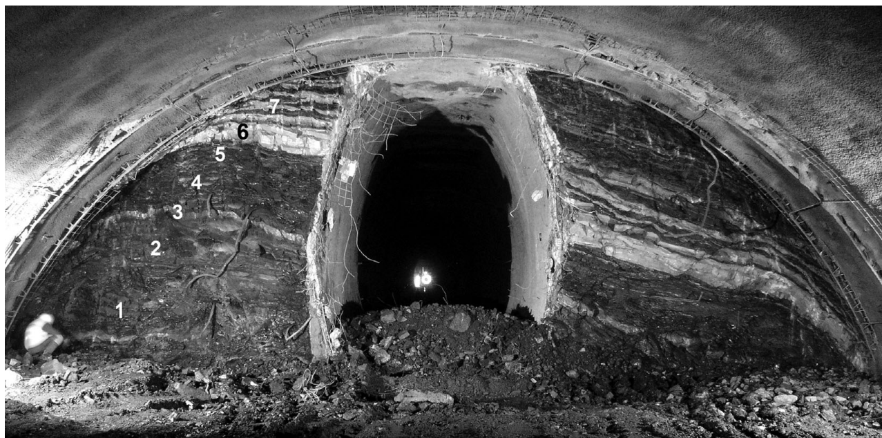
Figure 4. Middle Aeronian through to lowermost Telychian sedimentary rocks exposed in the face of the Radotín tunnel. No. 1 designates silty silicites and siliceous shales of the convolutus Zone, no. 2 points to pyrite-rich black shale of the lower sedgwickii Zone and no. 3 to a grey mottled silty bed in the middle part of the sedgwickii Zone. Micaceous black shale of the upper sedgwickii Zone is marked by no. 4. The black clayey shale (no. 5) immediately below the pale-coloured basal mudstone yielded graptolites of the rastrum Zone. The massive bed of pale-coloured, mottled carbonate mudstone, without graptolites, forms the base of the Litohlavy Fm. (no. 6). Lowermost Telychian graptolites of the linnaei Zone appear in the black claystone intercalations (no. 7) just above the basal mudstone. Photo by Jakub Bohátka.
