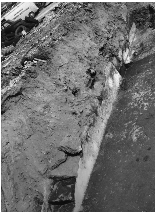
Fig. 13. Wall 4 viewed from the southwest (courtesy Soprintendenza).
