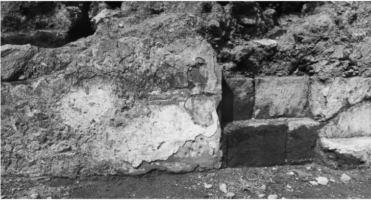
Fig. 15. Detail of wall 4 showing the different layers of plaster, viewed from the east (courtesy Soprintendenza).
