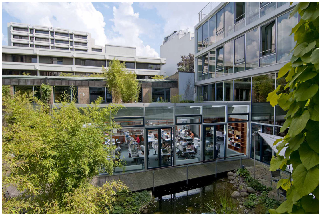
Figure 1. The Max Planck Institute building.
