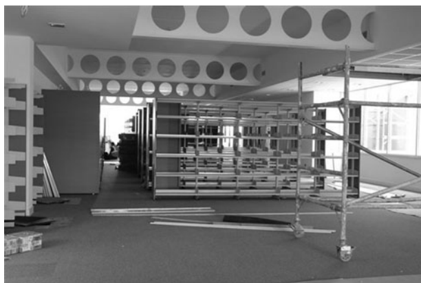
Figure 3: Library shelving construction.
