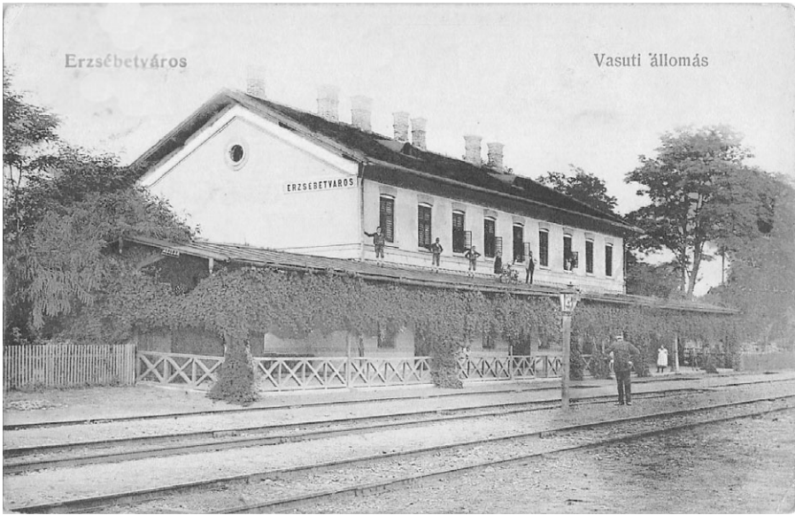
Figure 6. Dumbrăveni. First passenger building opened in 1873. View from the track side.
