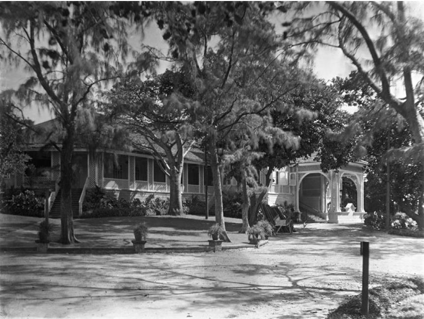
Figure 6: Government House, Malabar Point, Bombay, early twentieth-century view. Courtesy Bhau Daji Lad Sangrahalaya, Bombay.
