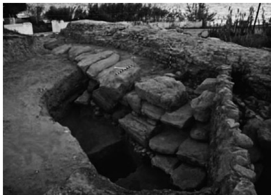
78. Mavra Litharia, ancient Aigeira: harbour mole. © Ministry of Education and Religious Affairs, Culture and Sports: 37 th EPCA.
