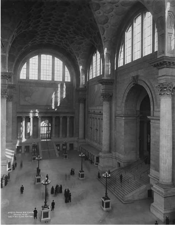
Fig. 5. Pennsylvania Station, entry hall and ticketing office, photograph of c. 1910 (New-York Historical Society)
