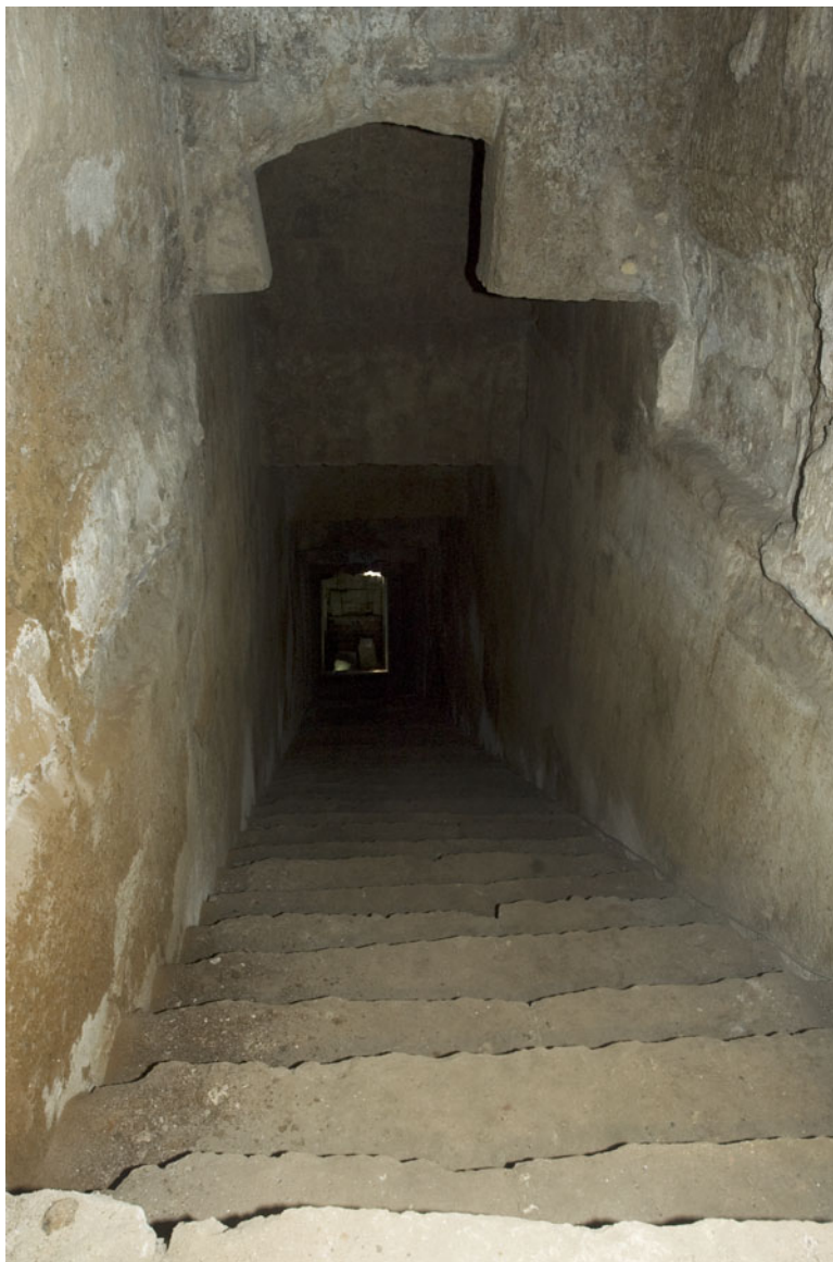
Fig. 11. Substructure on the Capitoline saddle, 78, stairs from the Forum Romanum to the Temple of Veiovis, and from the Temple of Veiovis to the summit. (© Penelope J.E. Davies).
