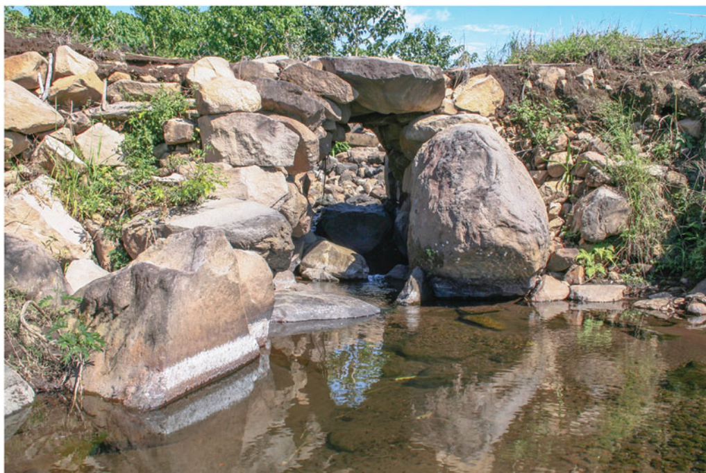
Figure 1. Thompson's bridge. Photograph taken from the south side, during the dry season in 2009, prior to the bridge's destruction (photograph by Oswaldo Chinchilla Mazariegos).
