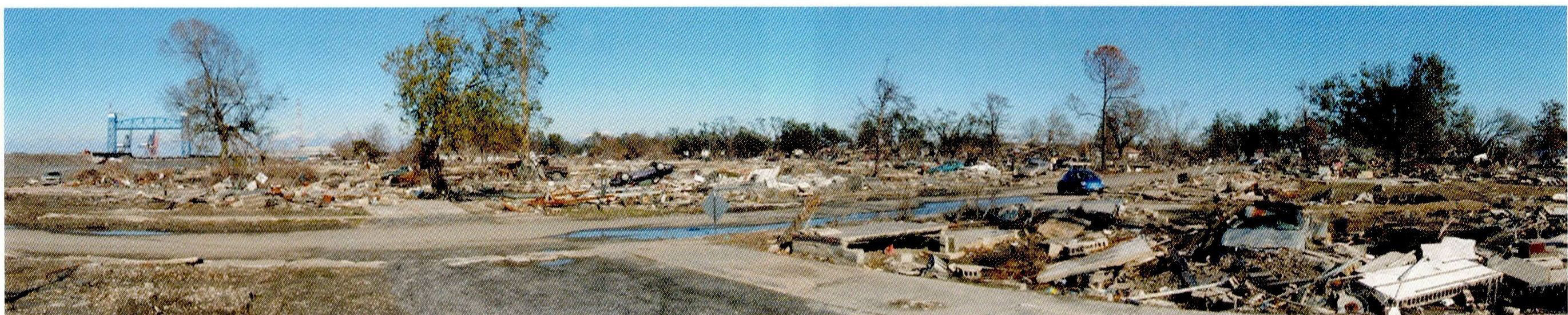
Fig. 5. Near-180° panoramic views in the immediate vicinity of breached levee sites in New Orleans. a. London Avenue Canal, with cranes on the righthand side indicating location of the breach where repairs are ongoing (see Fig. 2c). The open lot in front of the red crane was the location of the home that is in the centre of the panorama and was displaced ~40 m by the flood. Sediment-covered street on the lefthand side is oriented perpendicular to the canal. b. Outwash fan near the London Avenue Canal breach site with cranes on the lefthand side indicating location of the breach. The outwash fan consists predominantly of sands derived from the Pine Island barrier, a sand body that extends up to ~10 m below the surface (Saucier, 1963). Thickness of the fan is in places 1.5 m or more, sufficient to bury cars. Note the largest fan thicknesses in the wake of the remaining homes, separated by channel-like depressions between buildings (a more detailed discussion of this deposit is provided by Nelson & Leclair, 2006). Also note that roofs are nearly intact, testifying to the limited amount of wind damage compared to flood damage. c. Main breach in the Industrial Canal viewed from the Lower 9th Ward. The levee on the lefthand side has been almost completely restored. This area was built up with dense homes that were entirely eradicated. Note the nearly bare terrain near the breach site, giving way to piles of debris and overturned cars to the right. The radius of the area of complete destruction is at least ~400 m. Photos taken in December 2005.
