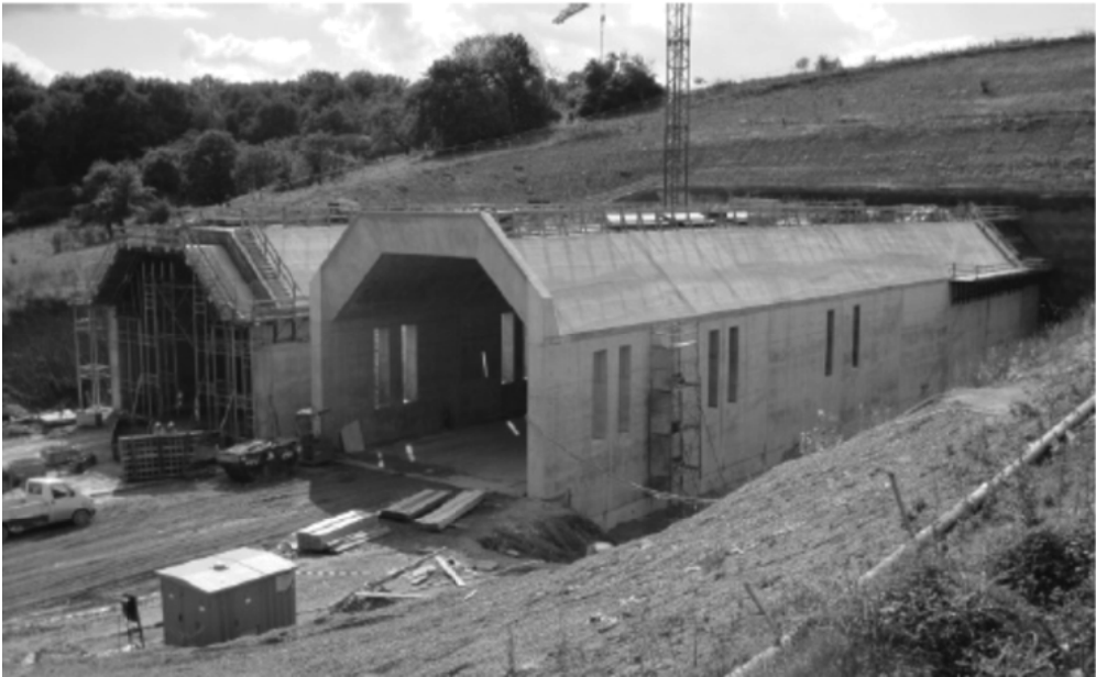
Figure 27. Construction of sonic boom alleviation section on the Finnetunnel tunnel in Germany (76) .
